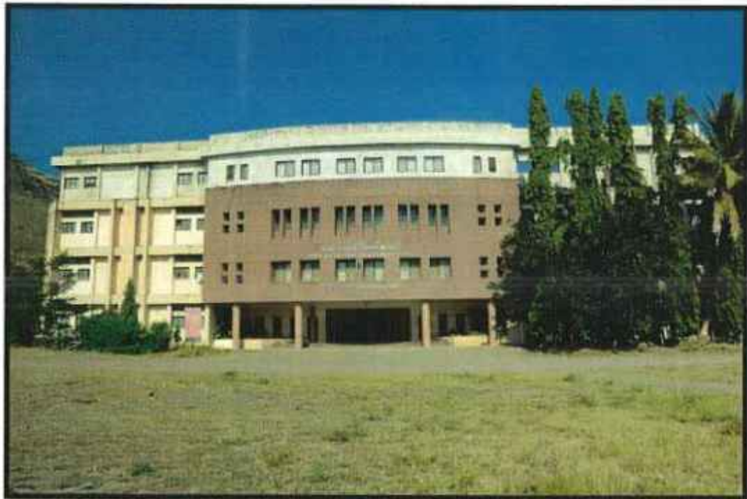
SSDJ College of Pharmacy 3 floor Building Front View
