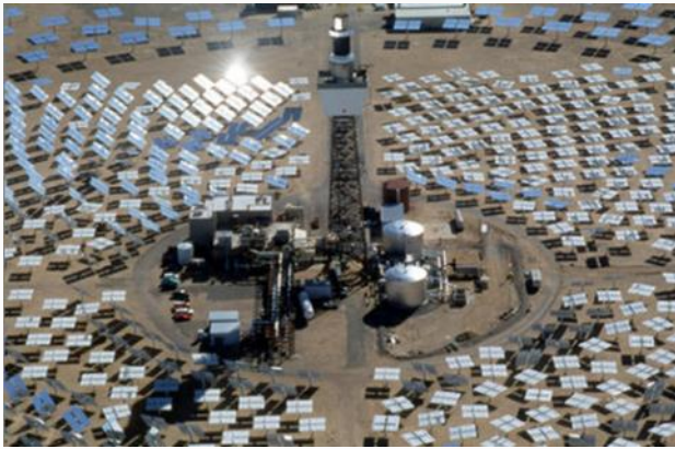
Fig.7. Solar Power Tower
